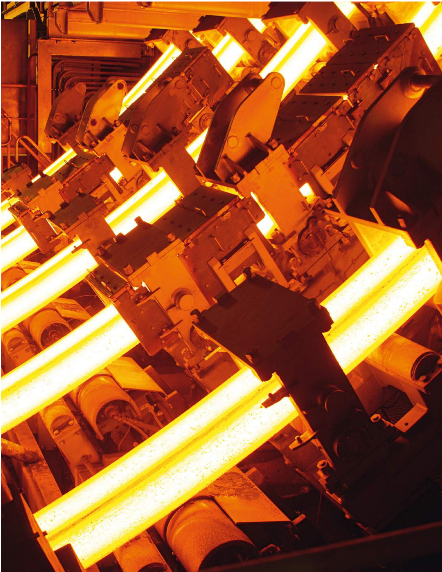
LD steelmaking plant Völklingen: Continuous casting plant
